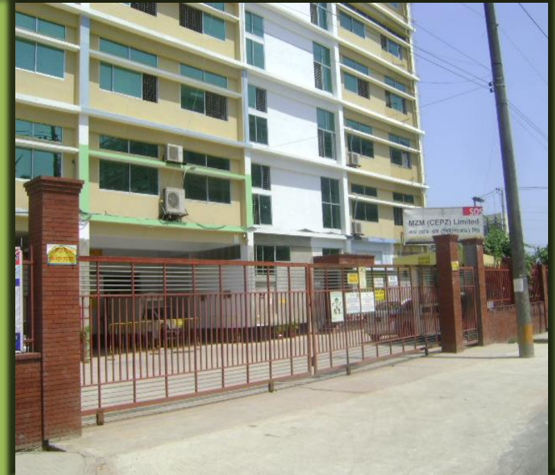
Factory Front Gate
