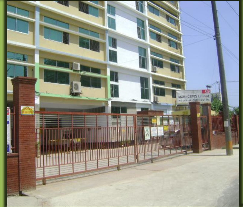
Factory Front Gate
