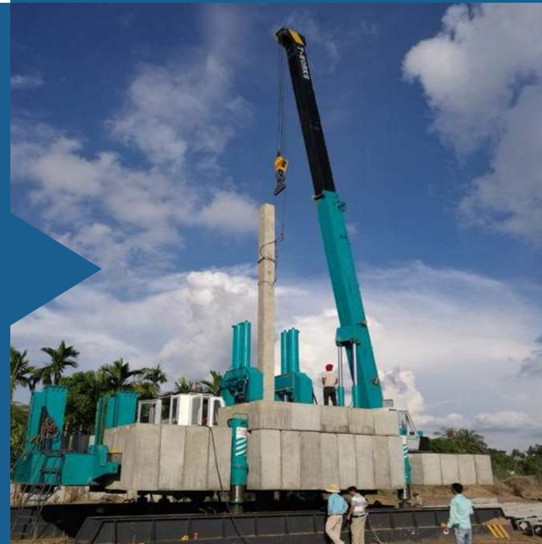
PICTURE OF 460MT HYDRAULIC PUSH HAMMER
