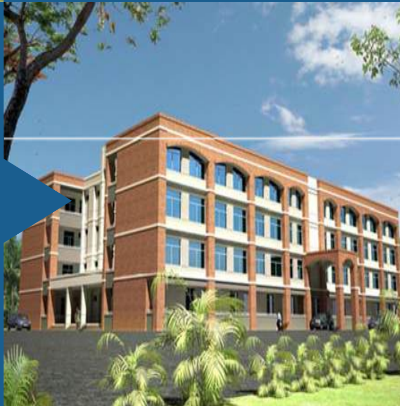
NARI PROJECT AT KEPZ, TRAINING COMPLEX, KEPZ, CTG.
