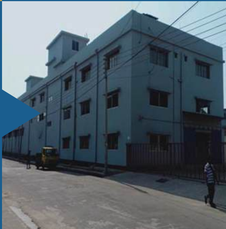
OFMA CAMP LTD. PADDING BUILDING . KEPZ, CHATTOGRAM
